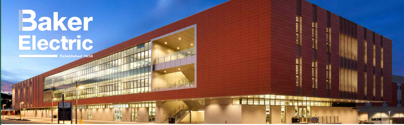
Photo Copyright © Baker Electric
