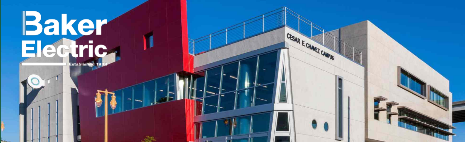
Photo Copyright © Baker Electric
