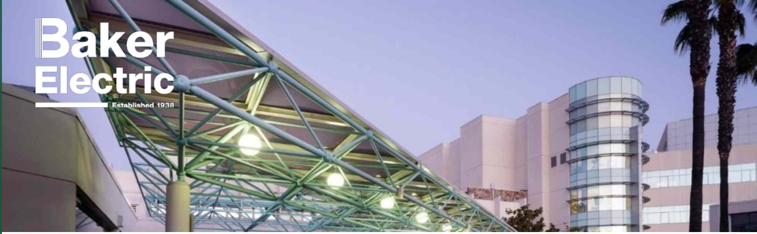
Photo Copyright © Baker Electric
