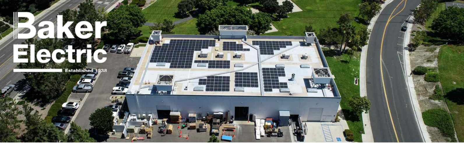
Photo Copyright © Baker Electric
