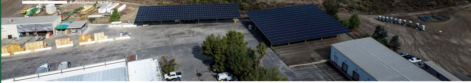
Photo Copyright © Baker Electric
