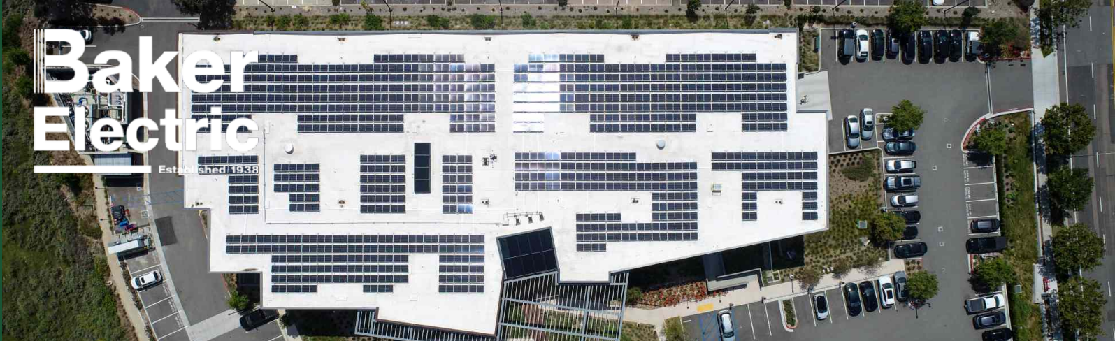
Photo Copyright © Baker Electric
