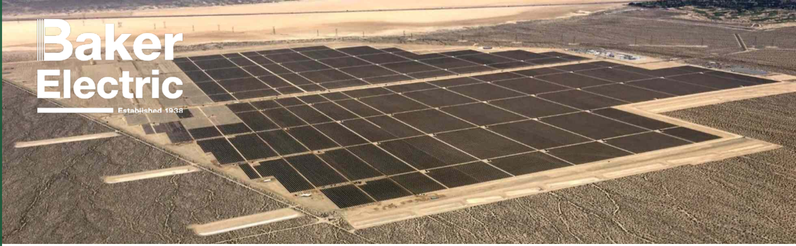
Photo Copyright © West Coast Aerial Photography, Inc.
